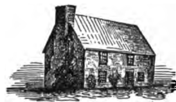
WHITFIELD HOUSE, AS SEEN FROM THE WEST.
